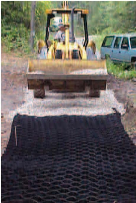
This photo shows a geotextile (or geoweb) installation. Technically a geotextile filter fabric is a synthetic material placed on the flat, under road fill. Its primary use is to keep layers separate, confine the road aggregate and to distribute the weight of the load.
